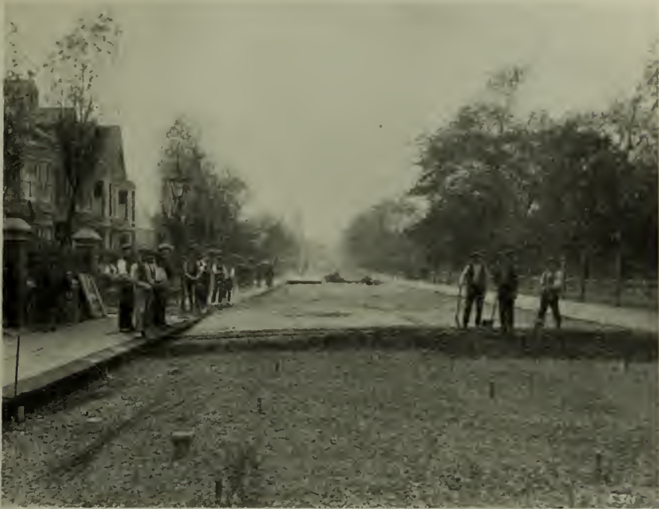
FIG. 14. SOUTHFIELD ROAD, MIDDLESBROUGH.
